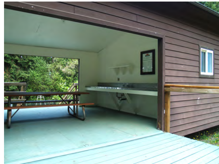
Picnic shelter/restrooms and wash area
