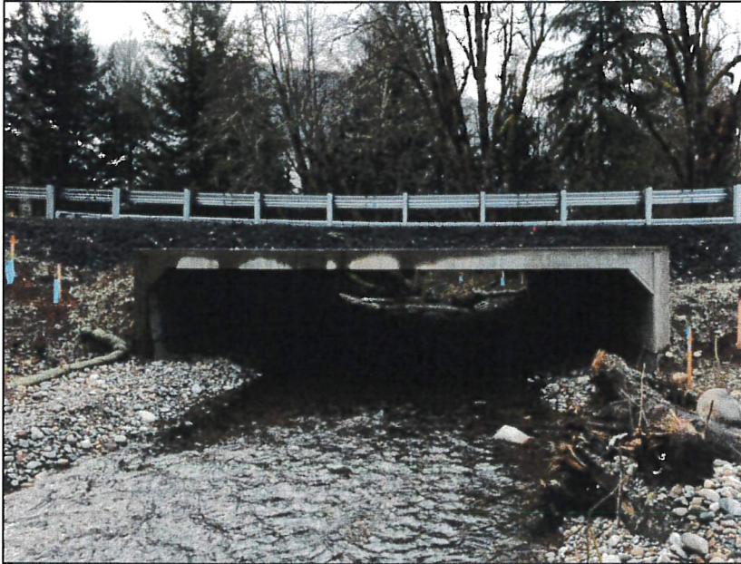
Crumb Rd MP 0.17, Bridge # 195 Post-Construction
