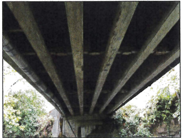
Hinning MP 0.23 Bridge #8
