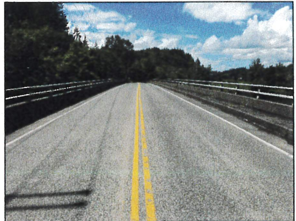
Galvin MP 1.55 Bridge #75
