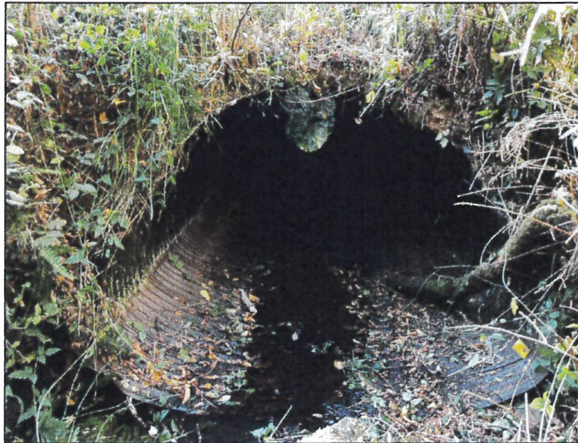
Centralia Alpha Rd MP 15.79, Bridge # 87 Pre-Construction
