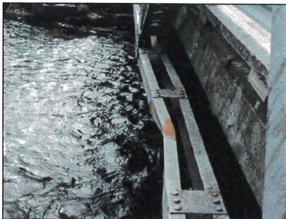
Davison MP 0.01 Bridge #1
