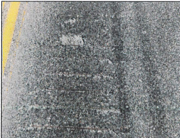
Galvin MP 1.55 Bridge #75
