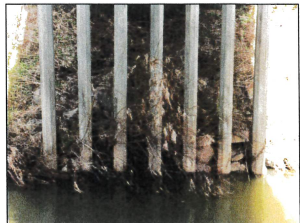
Wildwood MP 10.14 Bridge #3
