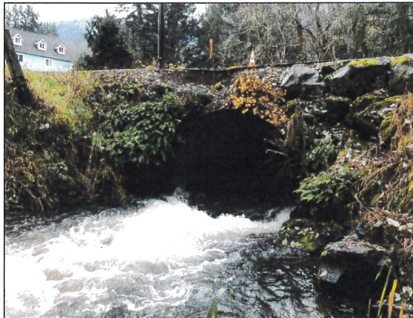
Crumb Rd MP 0.17, Bridge # 195 Pre-Construction
