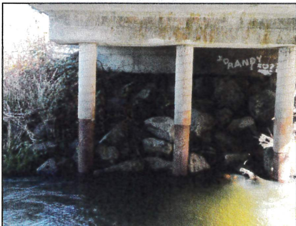
Senn MP 0.89 Bridge #77
