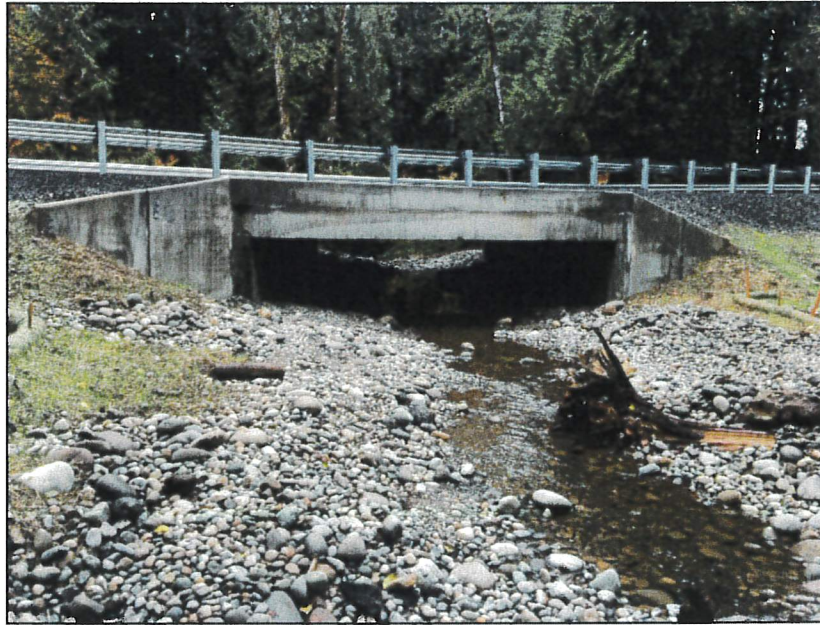
Centralia Alpha Rd MP 15.79, Bridge # 87 Post-Construction
