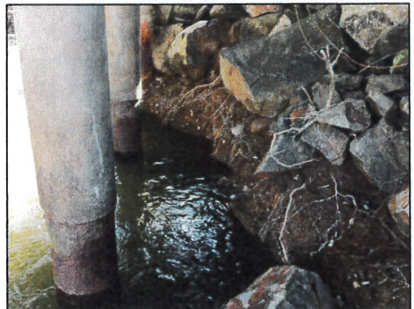
Senn MP 0.89 Bridge #77
