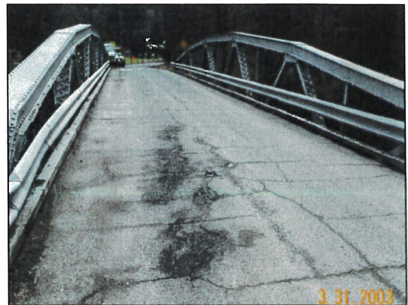
Davison MP 0.01 Bridge #1
