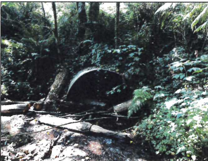
Lucas Creek Road MP 4.39 inlet
