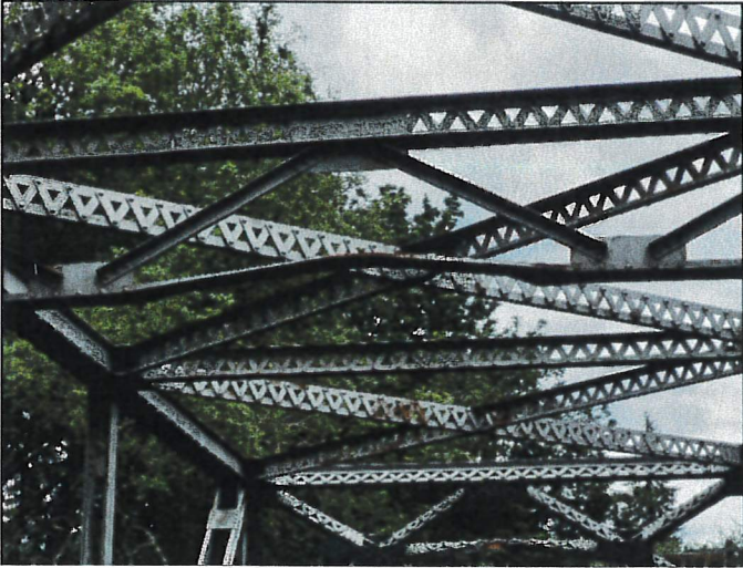
Ferrier Bridge #93 bent cross bracing
