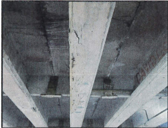
Hinning MP 0.23 Bridge #8
