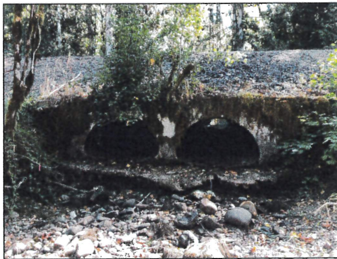
Kruger Road MP 1.20 outlet
