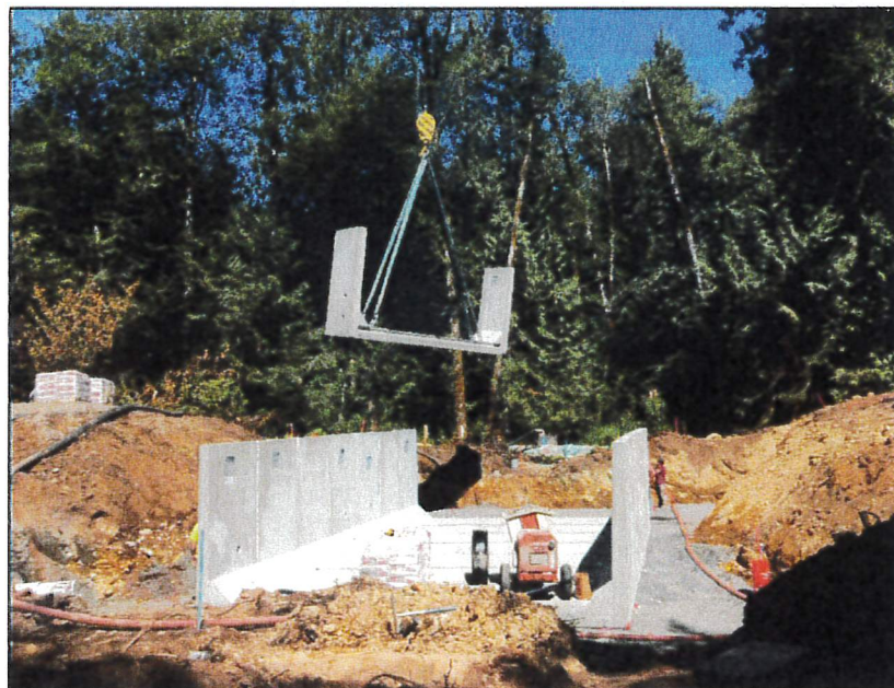
Centralia Alpha Rd MP 15.79, Bridge # 87 Mid-Construction
