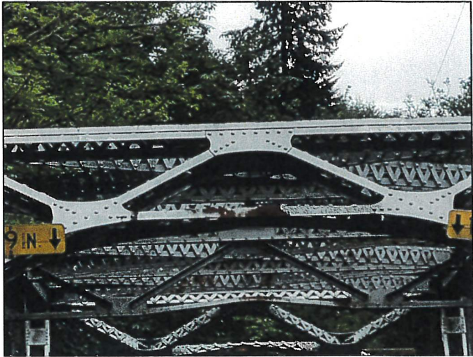
Ferrier Bridge #93 bent portal bracing
