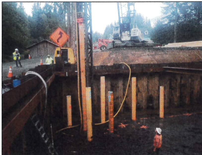
Crumb Rd MP 0.17, Bridge # 195 Mid-Construction
