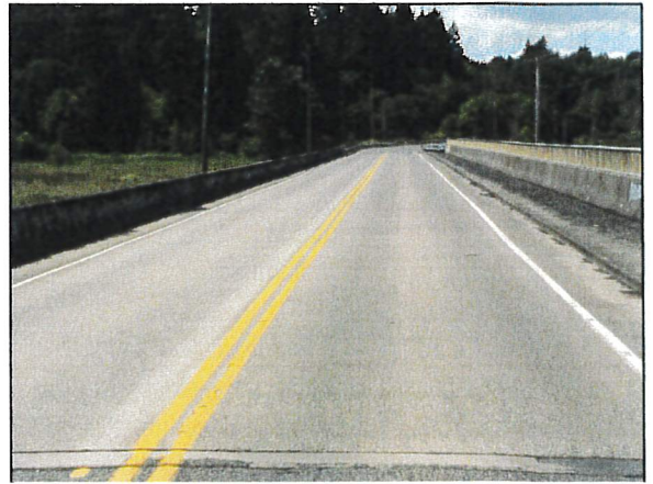
Galvin MP 1.23 Bridge #112
