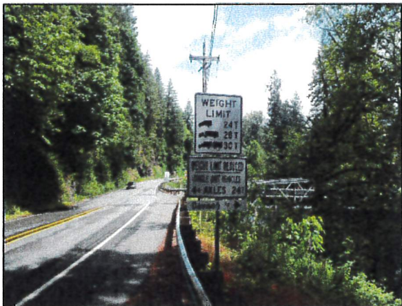
Davison Bridge #1 is posted with weight restrictions
