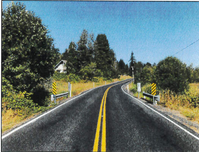
Logan Hill Road MP 0.10 roadway
