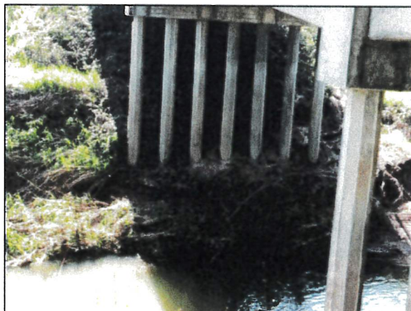
Wildwood MP 10.14 Bridge #3
