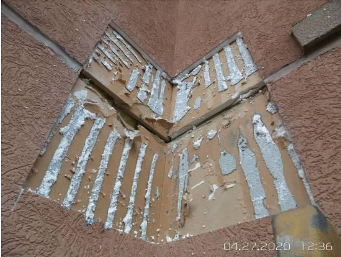
55. Opening 8 – no delamination or deterioration of the gypsum sheathing was observed.
