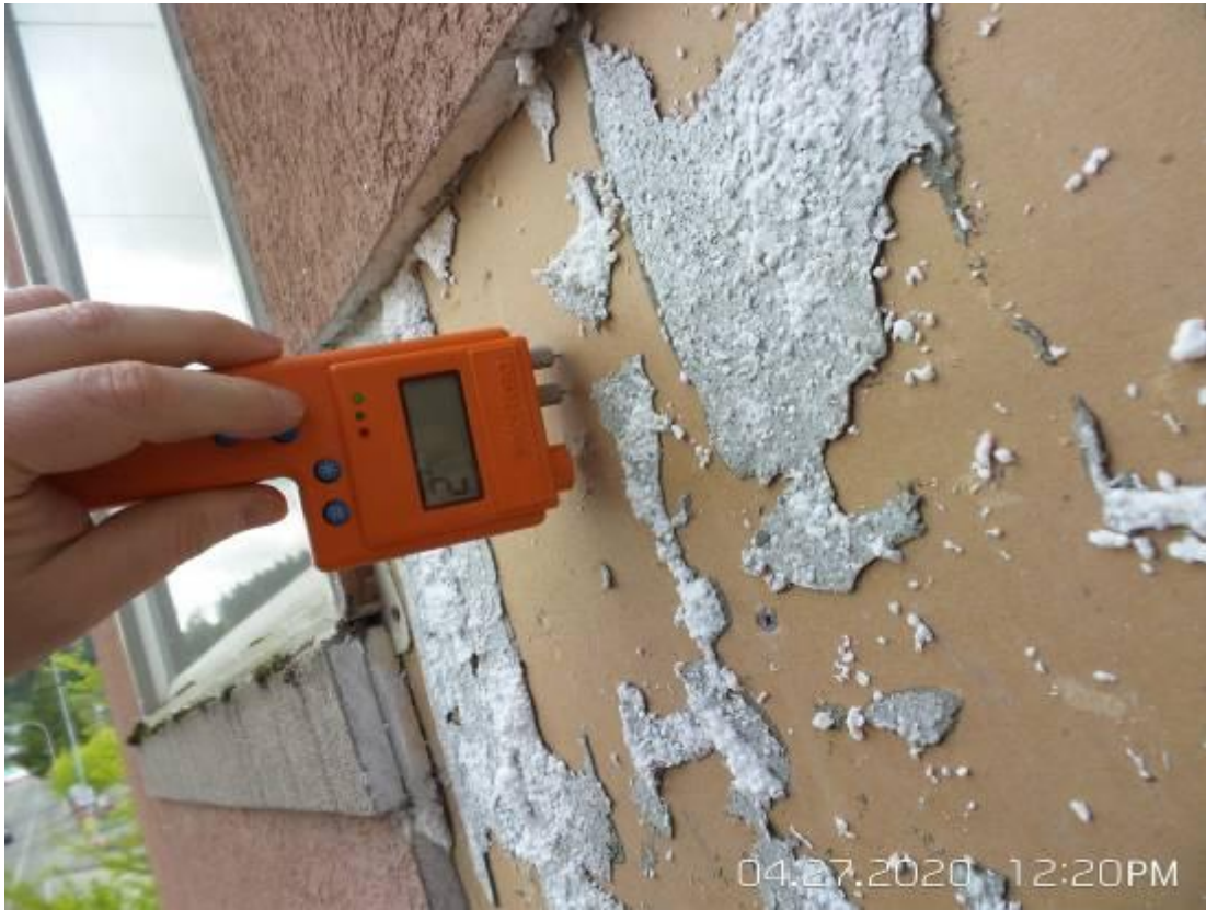
53. Opening 7 – moisture content readings of the gypsum sheathing were normal (0.1% - 0.2%).
