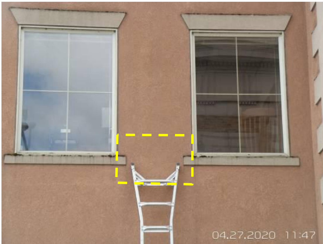
50. Opening 7 – remove cladding between windows.
