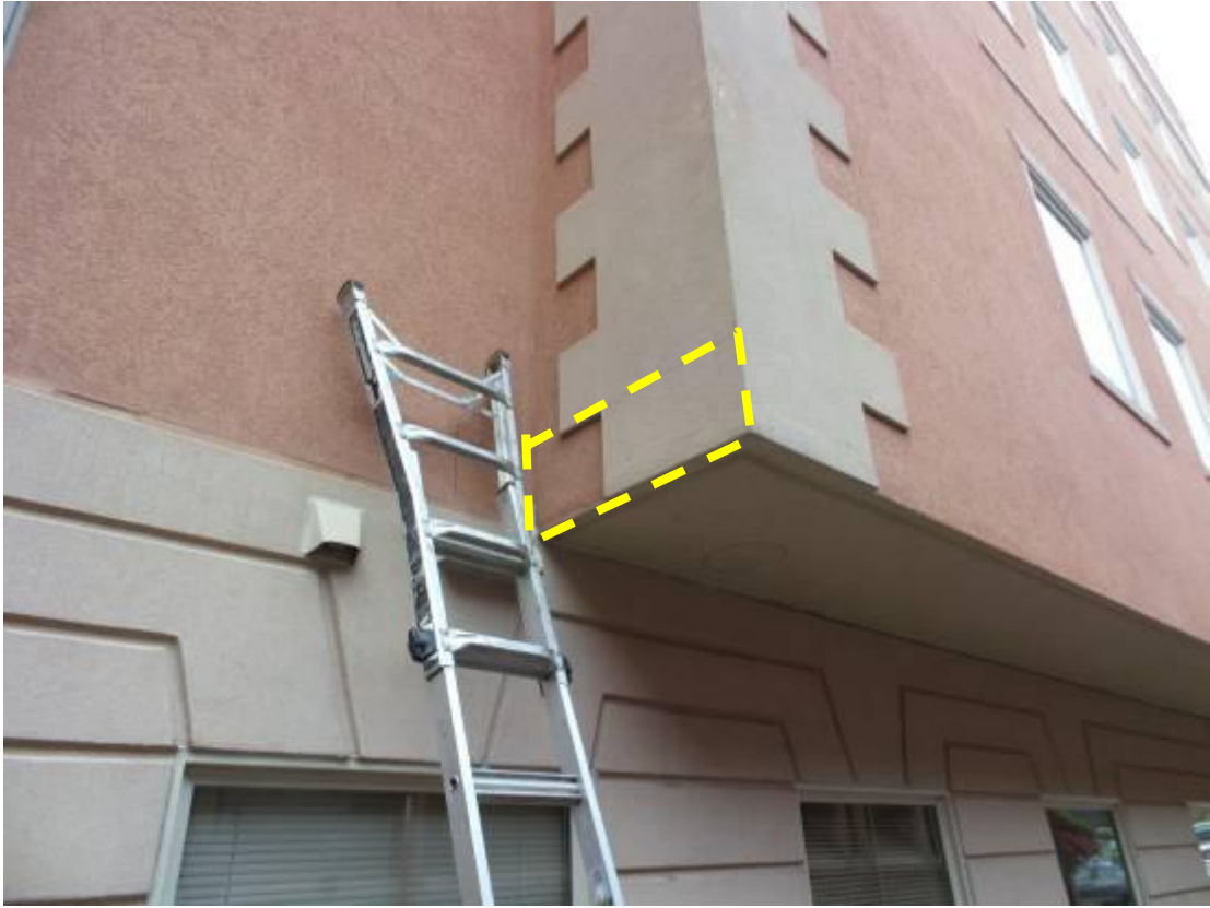
11. Opening 1 – remove cladding at inside corner above vents.
