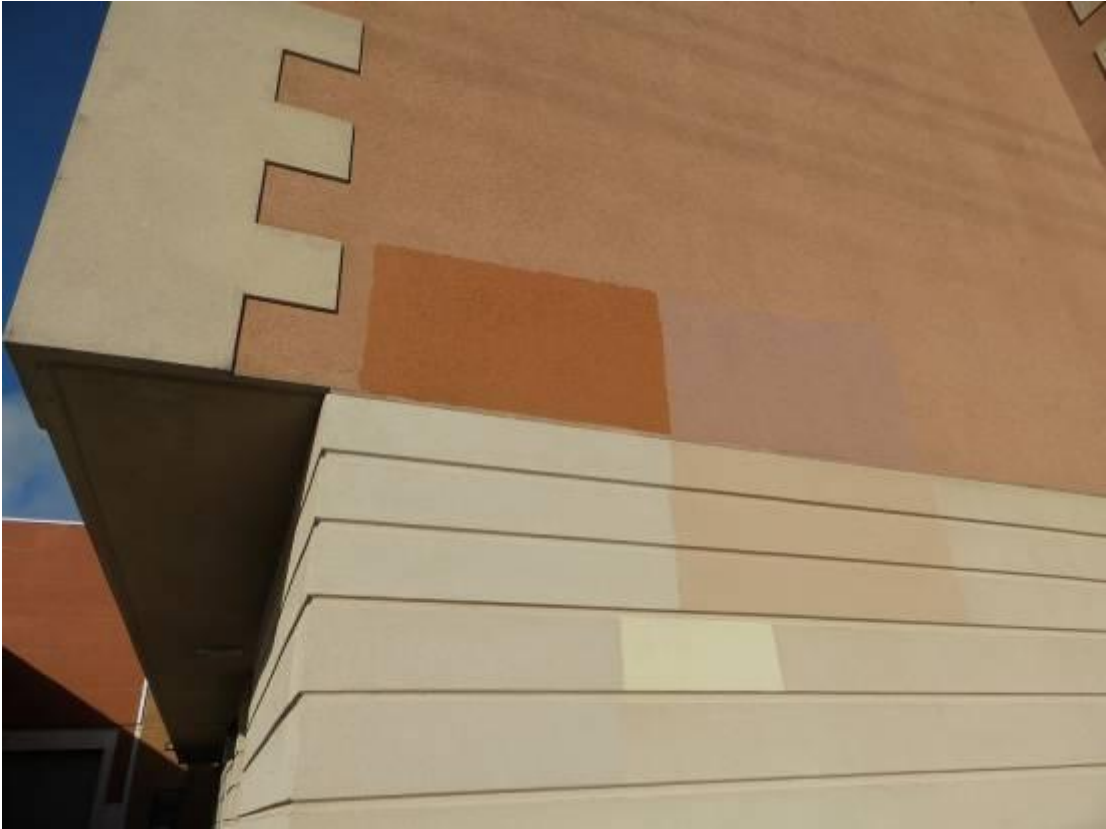
5. Original weathered finish with new test squares of paint for color selection.
