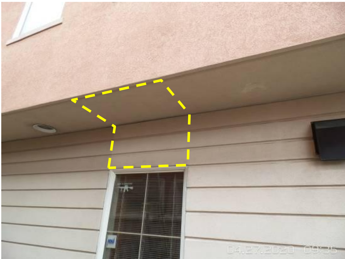
34. Opening 4 – remove cladding at window head and soffit.
