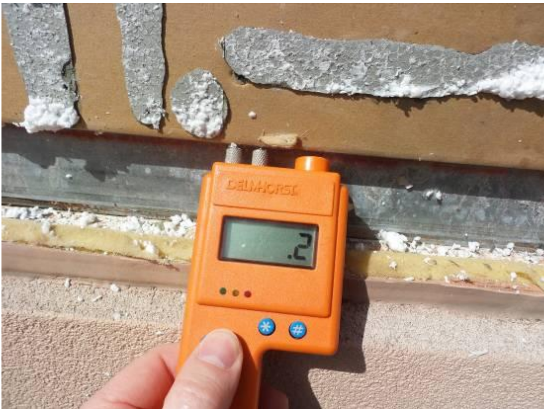
44. Opening 5 – moisture content readings of the gypsum sheathing were normal (0.1% - 0.2%).
