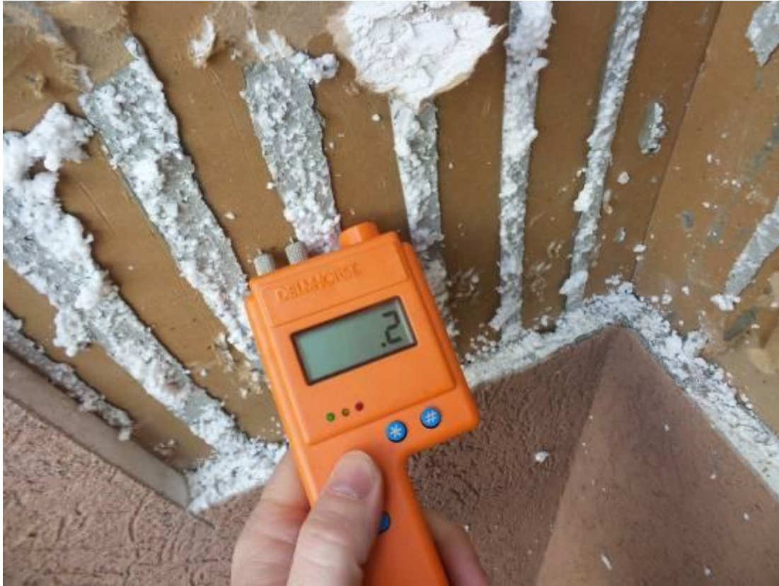
57. Opening 8 – moisture content readings of the gypsum sheathing were normal (0.1% - 0.2%).
