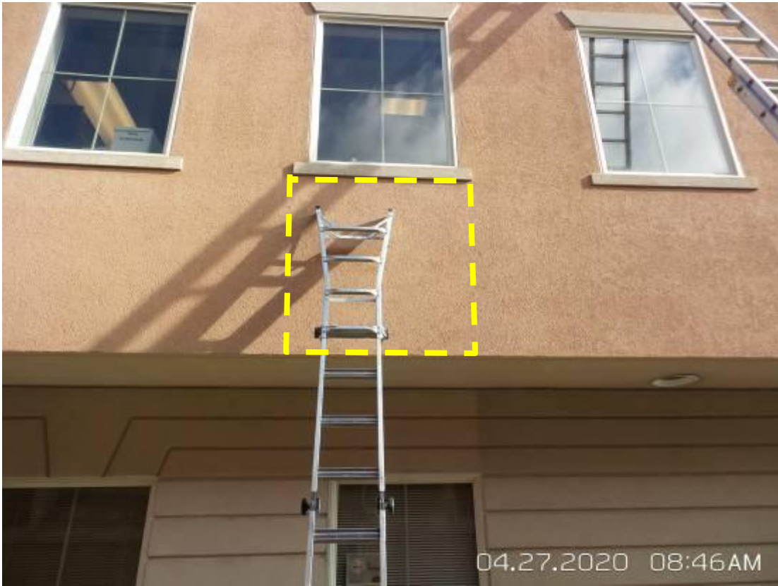
17. Opening 2 – remove cladding from window sill to soffit.
