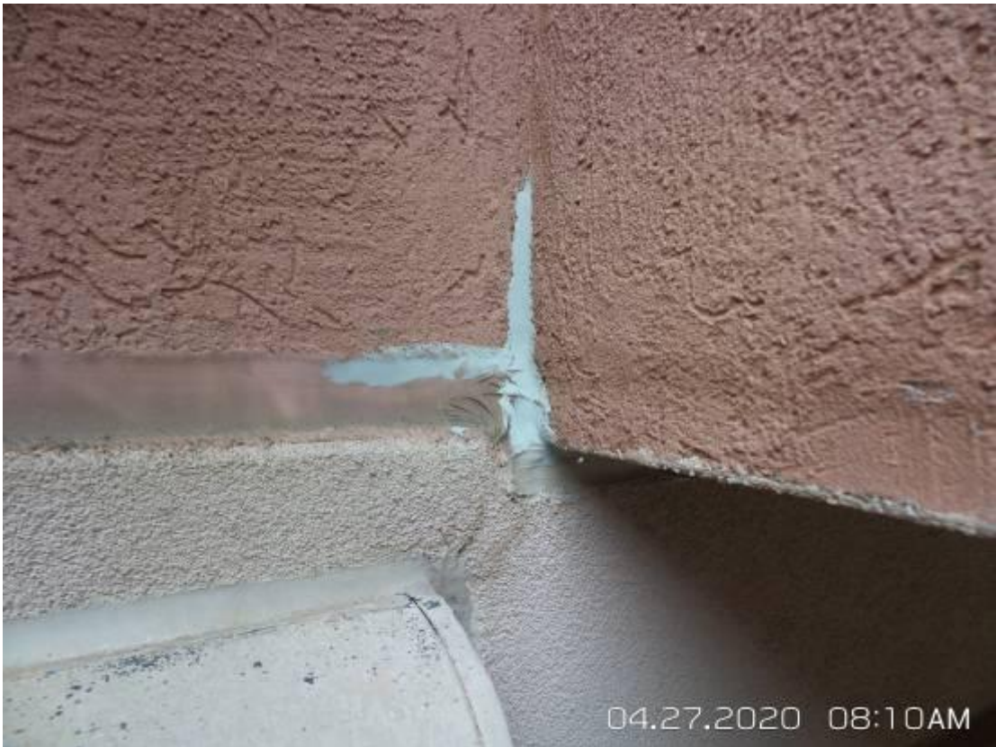
12. Opening 1 – new sealant observed at inside corner of wall and at wall to soffit intersection.
