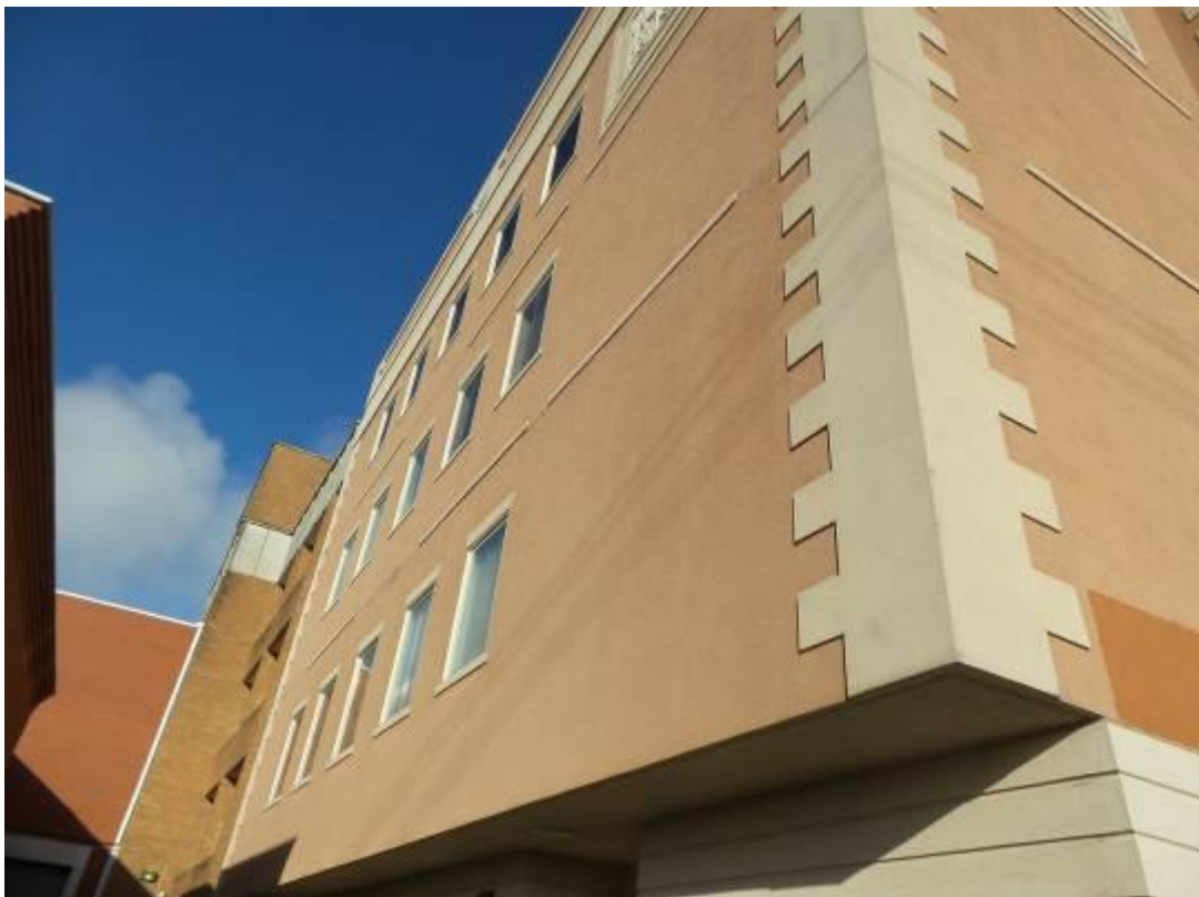
4. South elevation of courthouse addition circa 1995.
