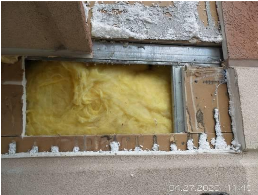
48. Opening 6 – gypsum sheathing was removed to observe the wall cavity.
