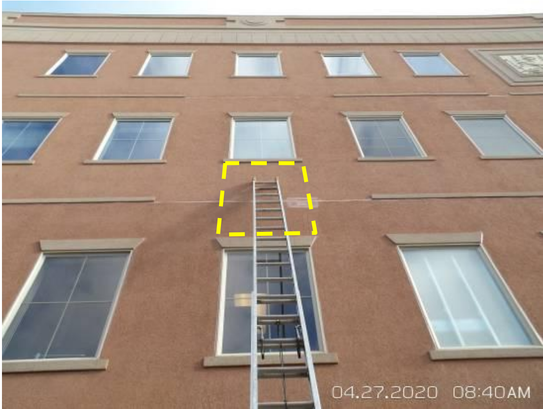
25. Opening 3 – remove cladding from third floor window sill to second floor window head.
