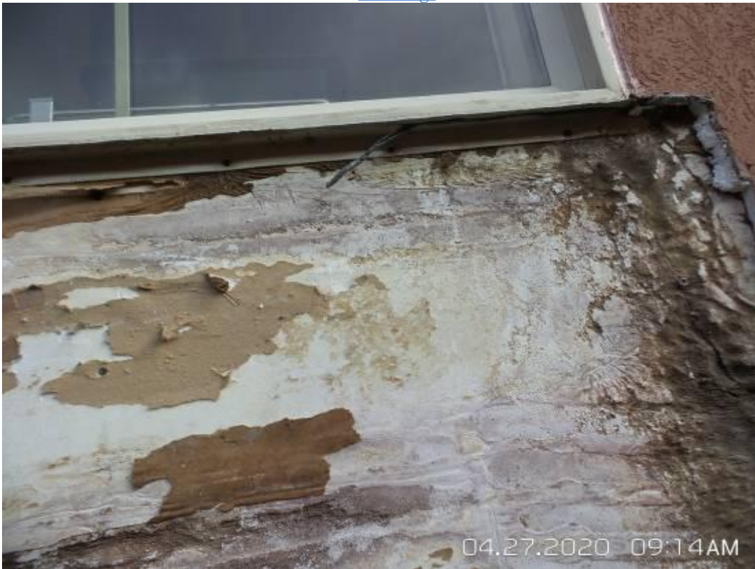
10. Vinyl framed flanged windows attached to steel through gypsum sheathing.
