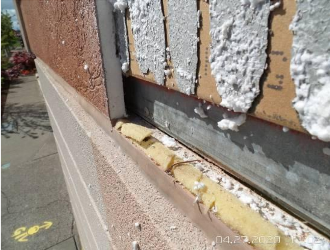
43. Opening 5 – no corrosion was observed on the steel stud framing.
