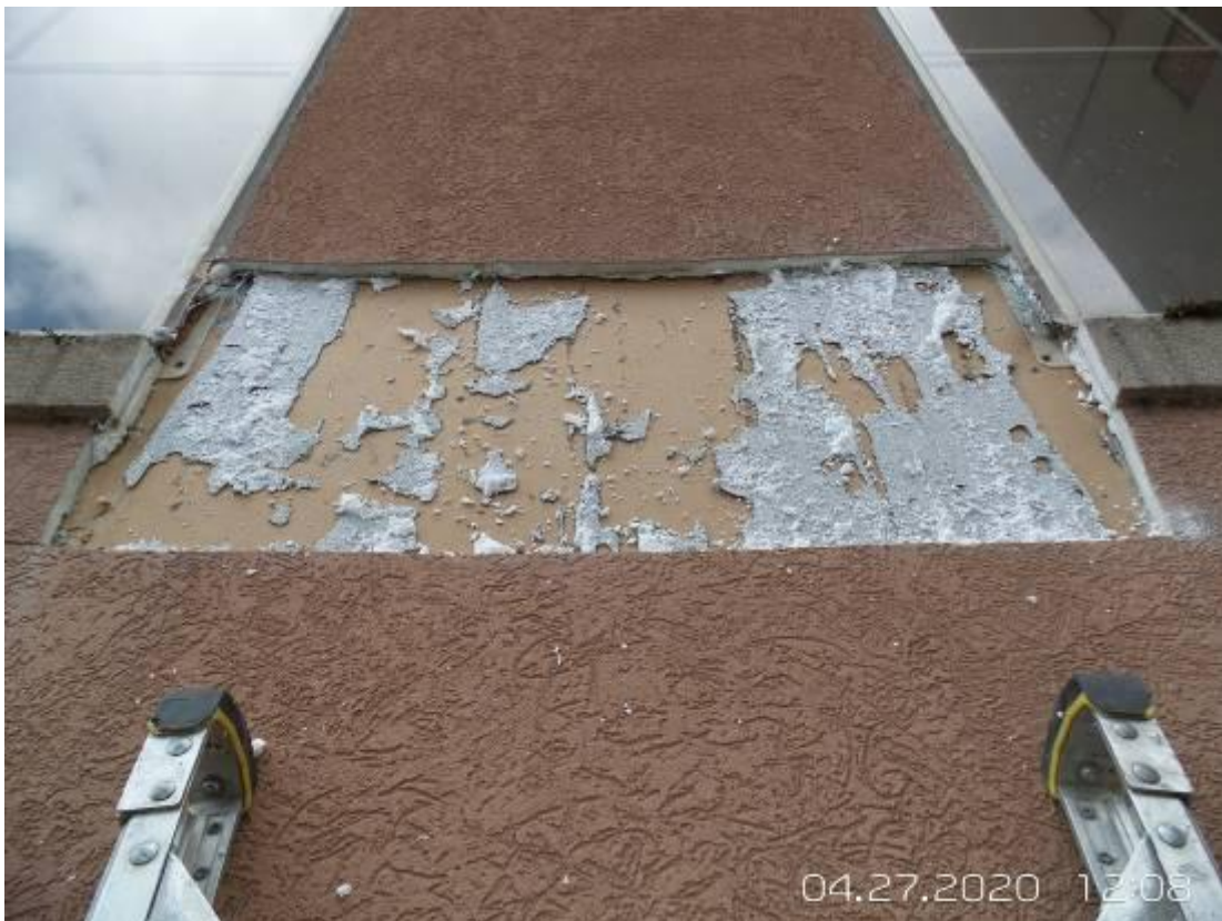
52. Opening 7 – delamination of gypsum sheathing was not observed.
