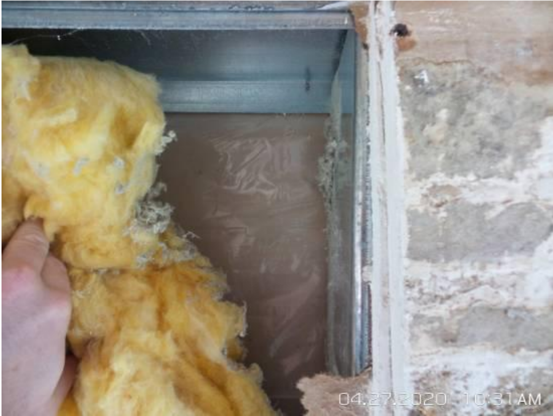
9. Insulation was non-faced fiberglass batt, and visqueen was installed on the interior of the steel stud framing.
