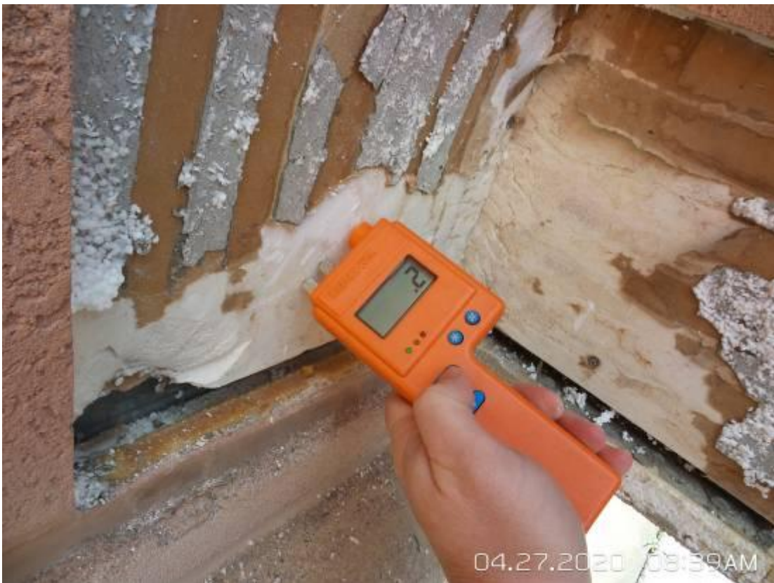
16. Opening 1 – moisture content readings of the gypsum sheathing were normal (0.1% - 0.2%).
