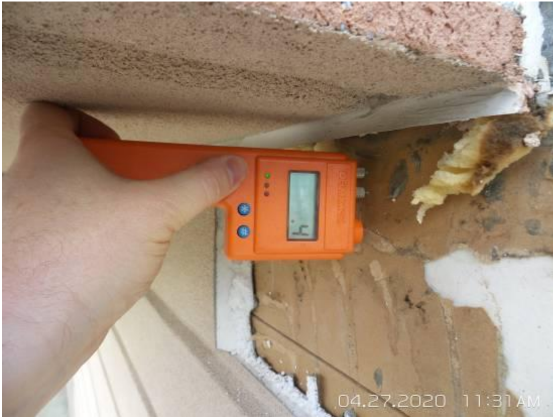
49. Opening 6 – moisture content readings of the gypsum sheathing was normal (0.2% - 0.4%).
