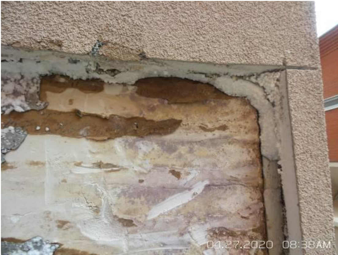
15. Opening 1 –the gypsum sheathing was stained at the outside corner of opening.
