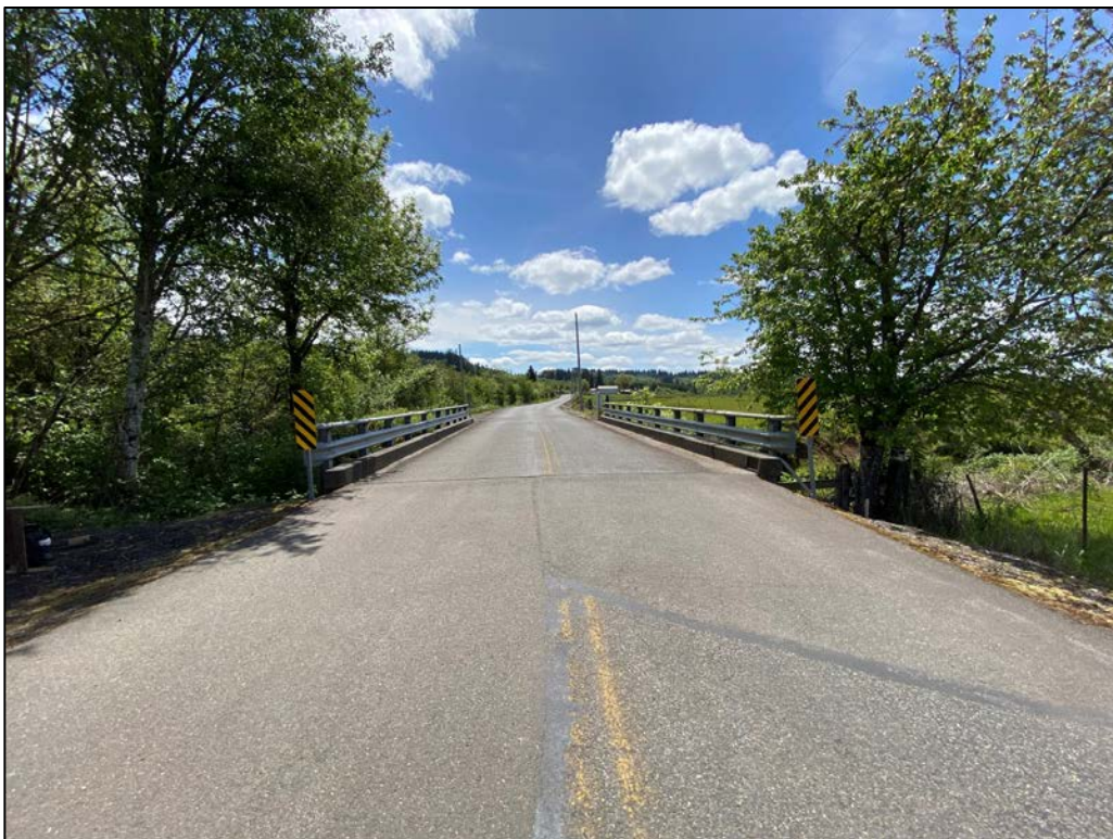
Figure 19. Overview of the Senn Road and Senn Bridge. View to the south.
