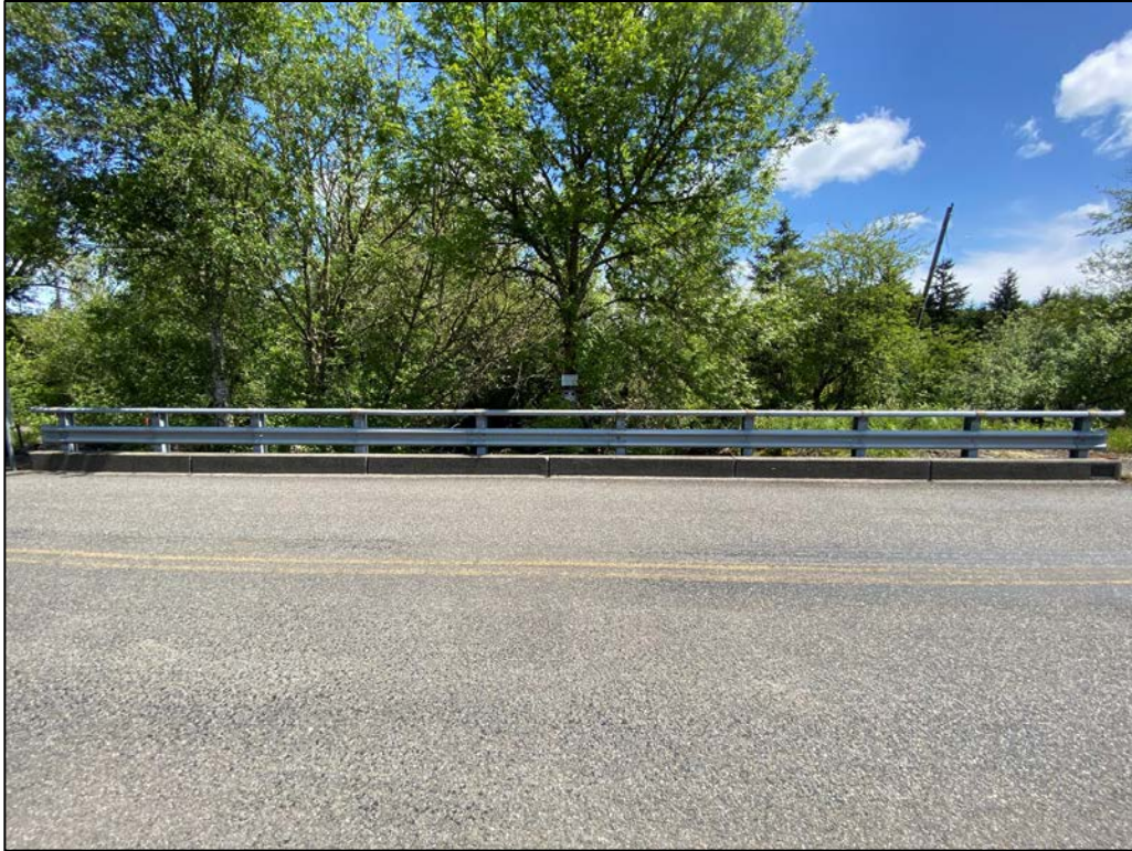
Figure 16. Overview of the eastern half of the project and Senn Bridge. View to the east.
