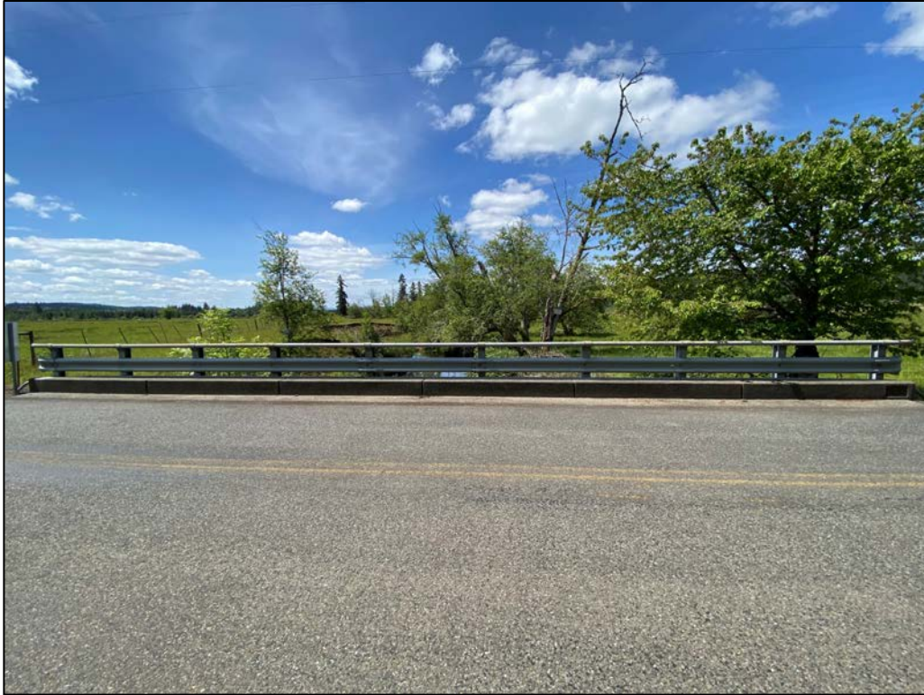
Figure 10. Overview of the western half of the project. View to the west.
