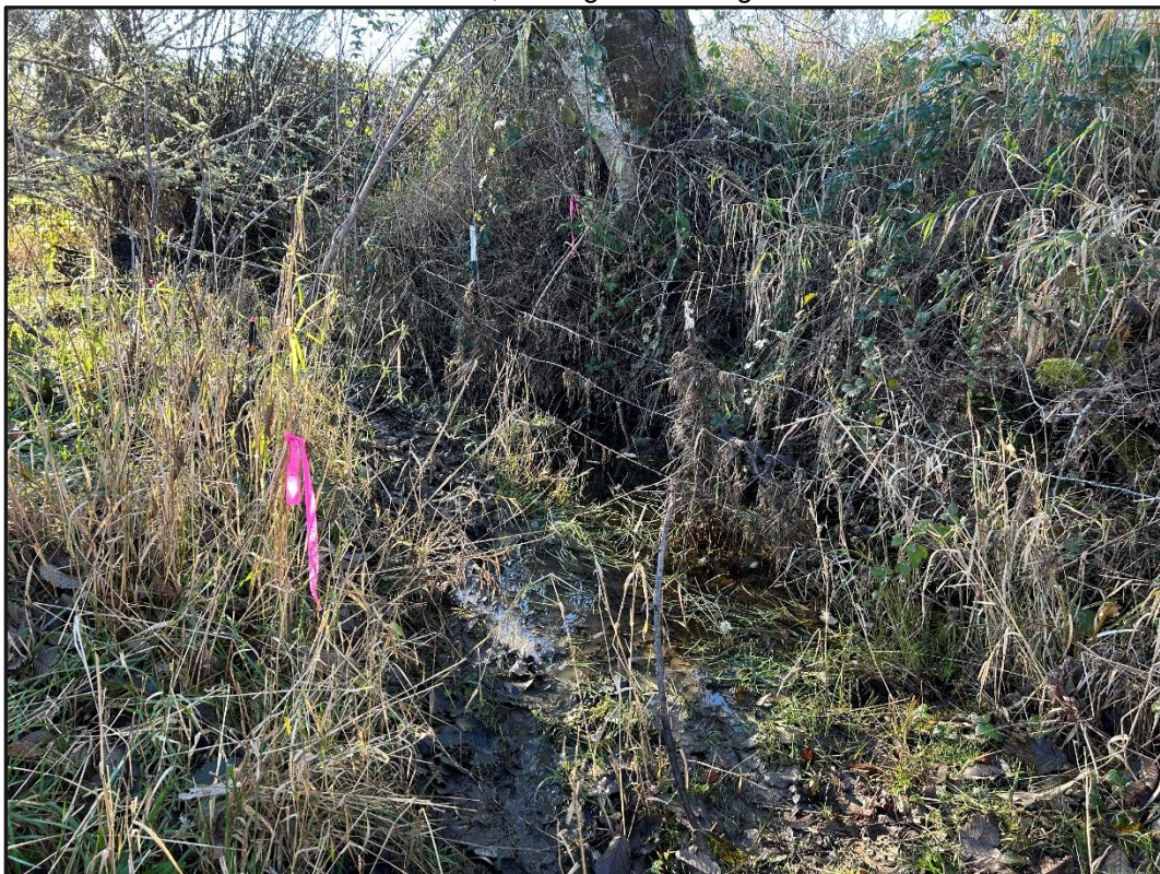
4. Typical conditions in Wetland 4, looking west toward Senn Road
