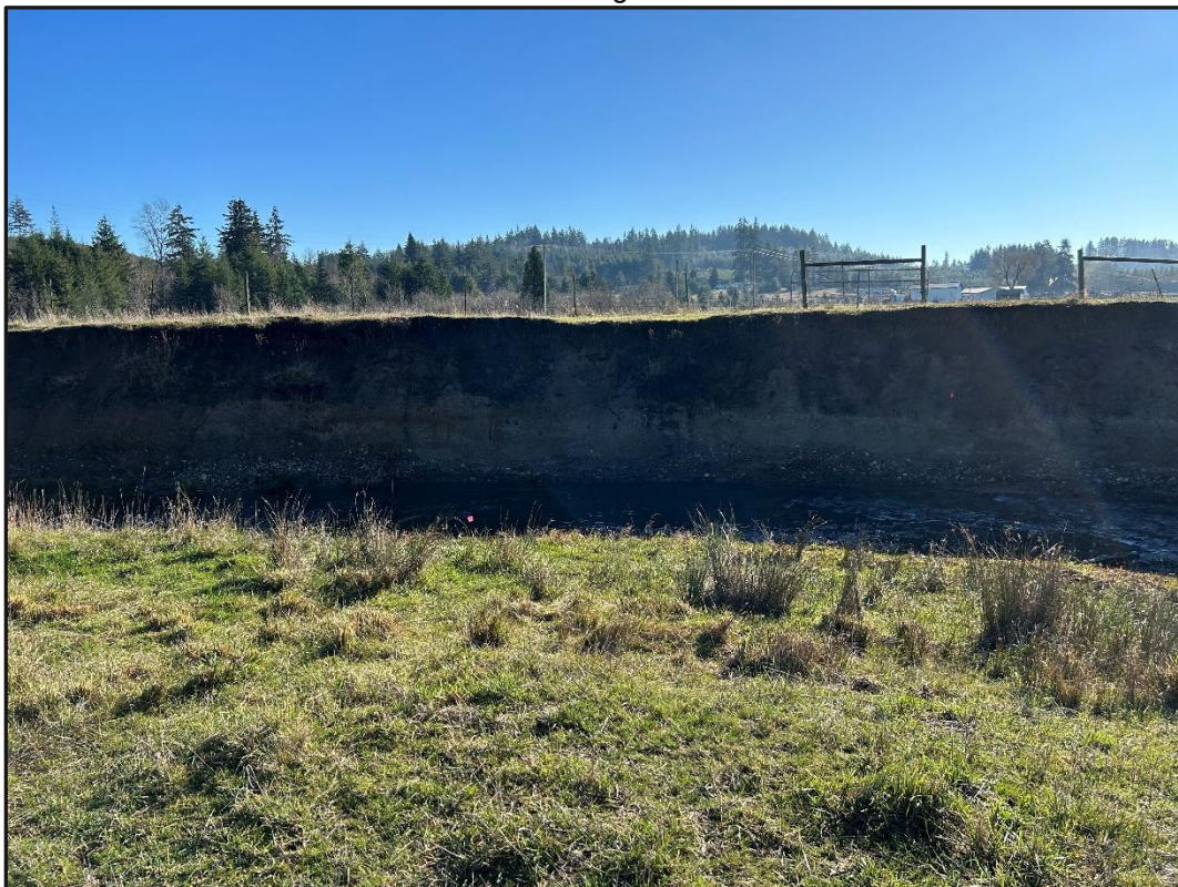
10. Typical erosion along south bank of Lucas Creek west of Senn Road.
