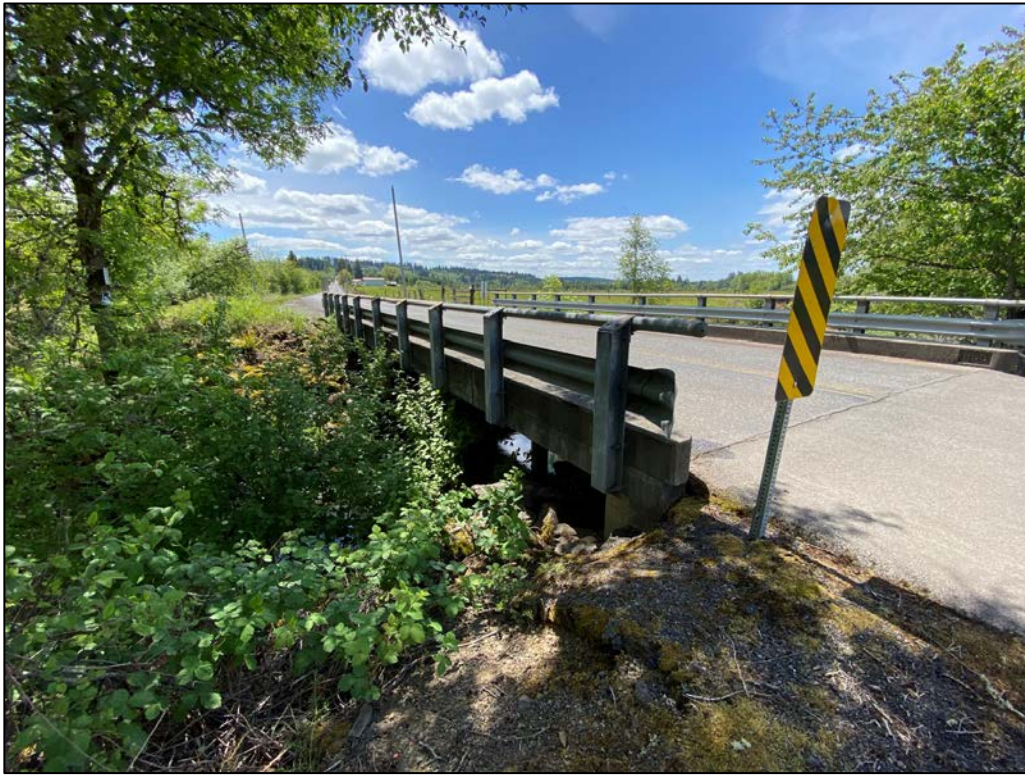
Figure 20. Overview of the Senn Road, Senn Bridge, and Lucas Creek. View to the southwest.
