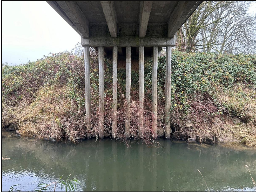
3. North bank of South Fork Chehalis River and piles of Lewis County Bridge No. 03, viewed from south bank
