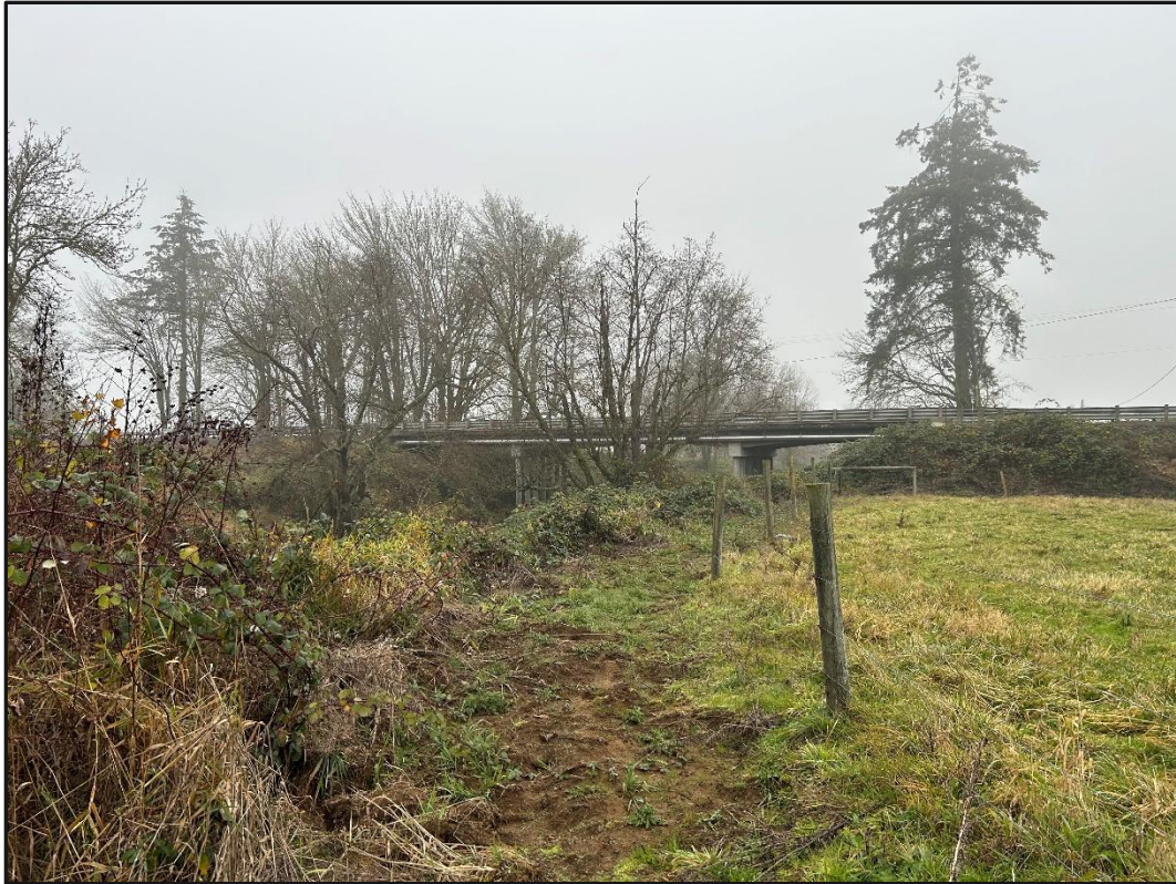
7. Top of south bank of South Fork Chehalis River looking east toward Lewis County Bridge No. 03 with livestock fields to the south
