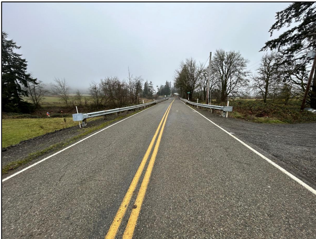
10. Wildwood Road and Lewis County Bridge No. 03 looking north
