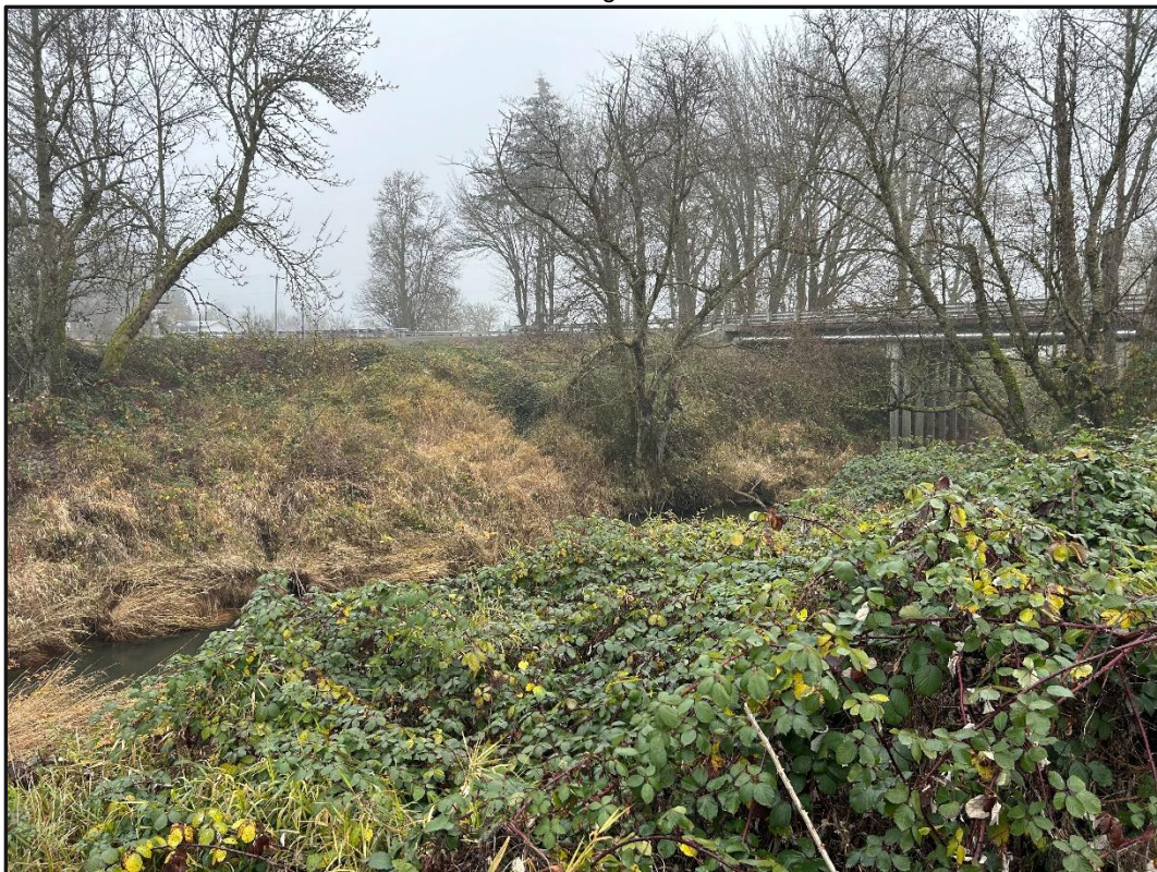
6. South Fork Chehalis River and Lewis County Bridge No. 3 looking northeast from the top of the south bank
