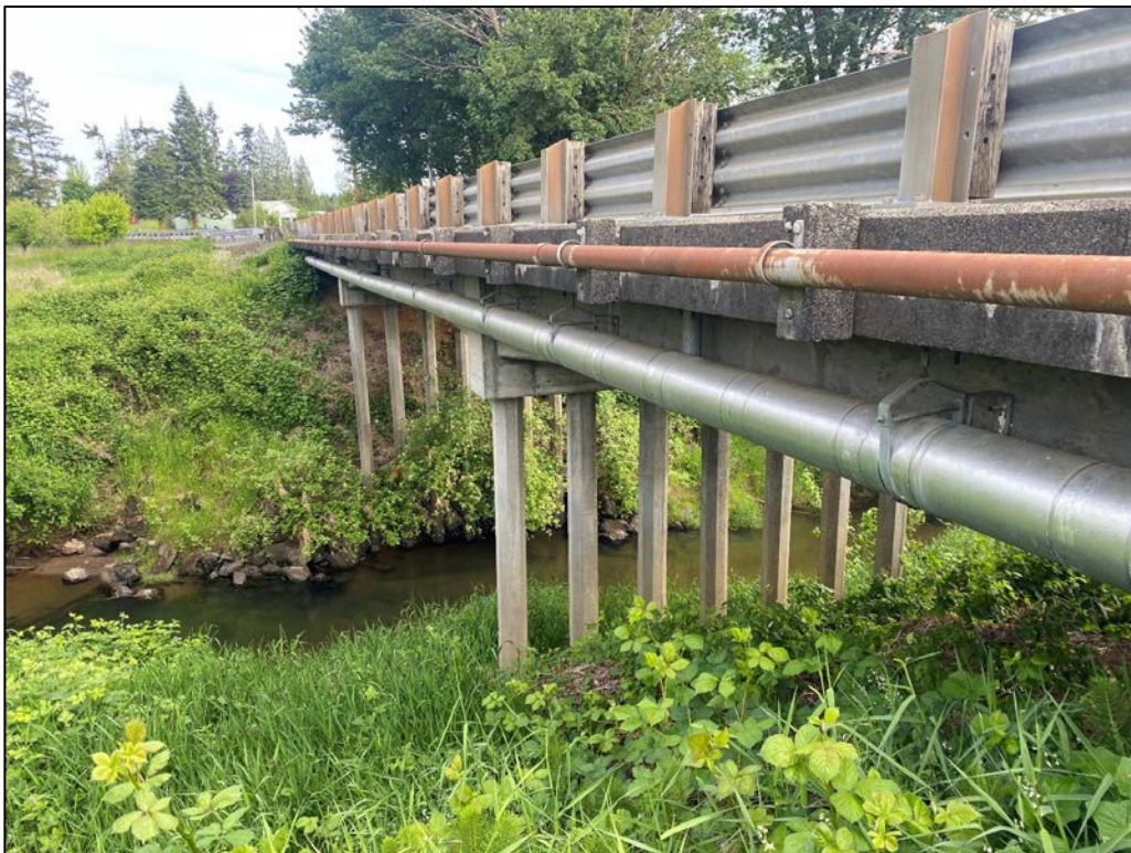
Figure 15. Overview of the South Fork Chehalis River and bridge in the vicinity of probe #5. View to the northeast.
