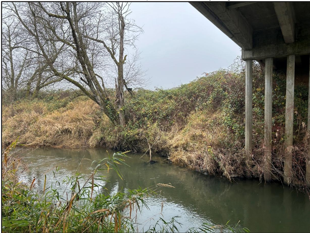
4. North bank of South Fork Chehalis River and piles of Lewis County Bridge No. 03, viewed from south bank
