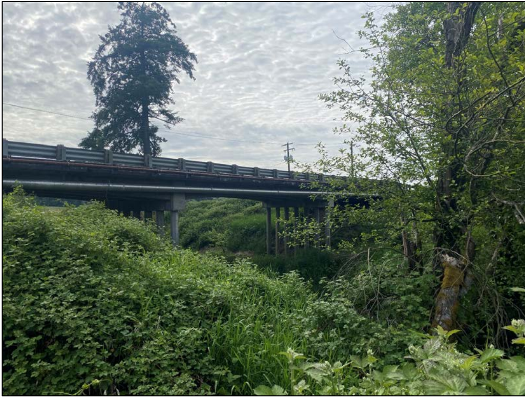
Figure 16. Overview of the Wildwood Bridge in the vicinity of probe #2. View to the southeast.
