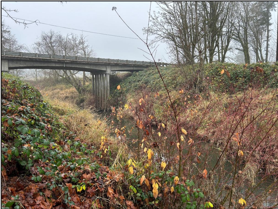
2. Lewis County Bridge No. 3 and the South Fork Chehalis River, looking west from south bank of South Fork Chehalis River
