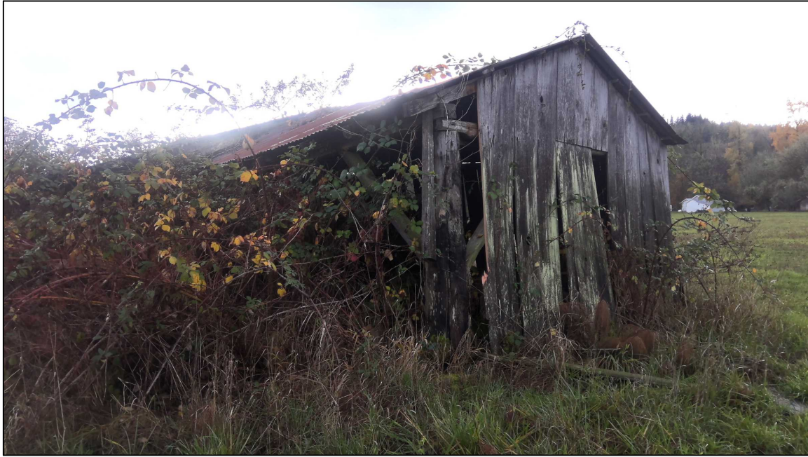
FIGURE 9--EXISTING STORAGE SHED DEMLISHED JANUARY 2026. PHOTO DATED 11-13-25
