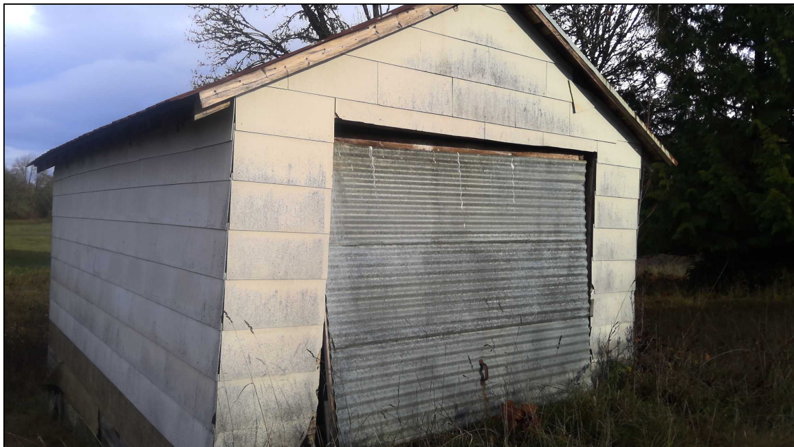
FIGURE 2--EXISTING GARAGE/ STORAGE SHED. DEMOLISHED JANUARY 2026.
