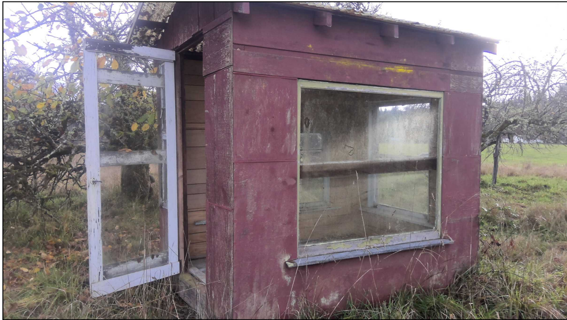
FIGURE 3--EXISTING SHED TO BE DEMOLISHED. PHOTO DATED 11-13-25. DEMOLISHED JANUARY 2026
