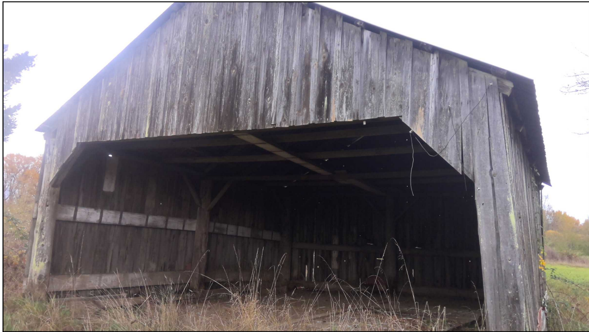
FIGURE 7--EXISTING MACHINE SHED. DEMOLISHED JANUARY 2026. PHOTO DATED 11-13-25
