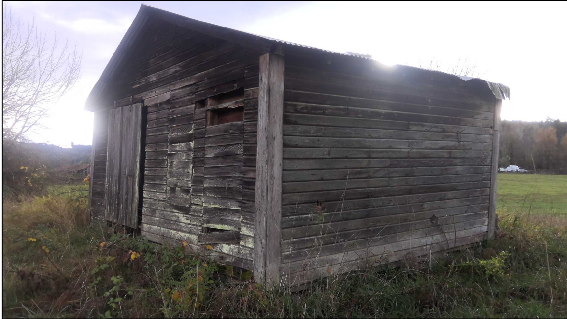
FIGURE 5--EXISTING GRANARY DEMOLISHED JANUARY 2026. PHOTO DATED 11-13-25
