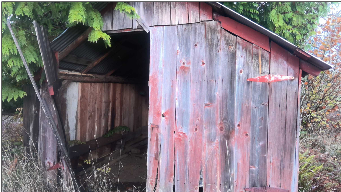
FIGURE 4--EXISTING STORAGE SHED. DEMOLISHED JANUARY 2026
