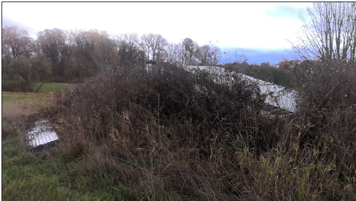
FIGURE 8--COLLAPSED EXISTING STORAGE SHED. DEMOLISHED JANUARY 2026
