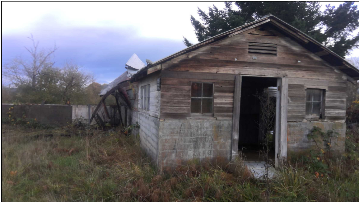
FIGURE 6--EXISTING CREAMERY/STORAGE SHED. DEMOLISHED JANUARY 2026
