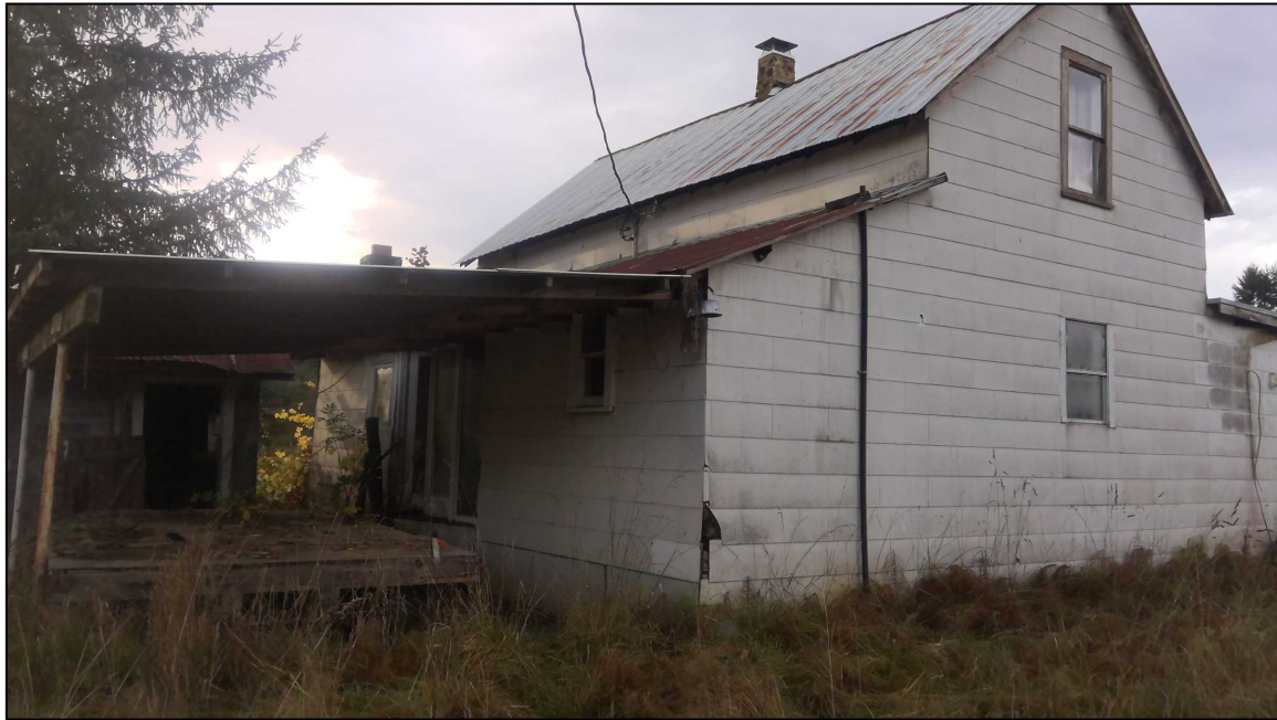
FIGURE 1--EXISTING RESIDENCE CONSTRUCTED CA. 1900. DEMOLISHED JANUARY 2026. PHOTO DATED 11-13-25
