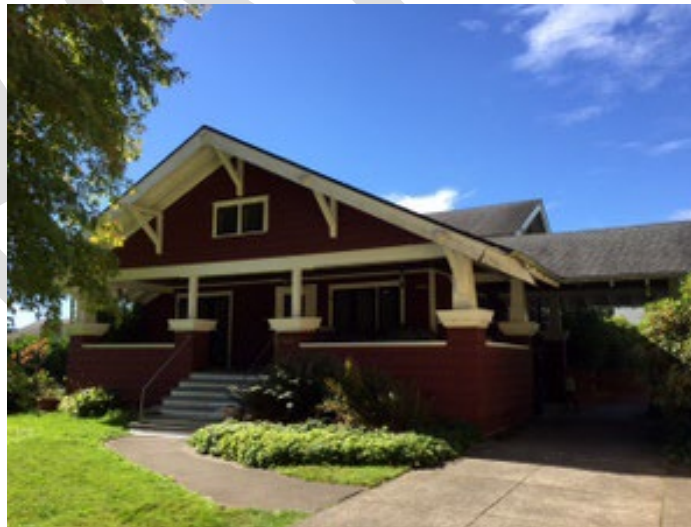
Onalaska Home built by Carlist Lumber Company est. 1915
