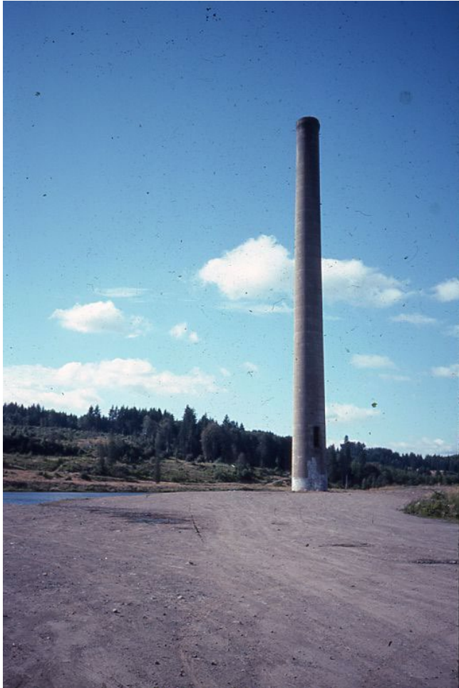
P23829 - Carlise Mill, Onalaska, WA Employed 1000, 1914-1942. Smokestack is 225 ft high.
