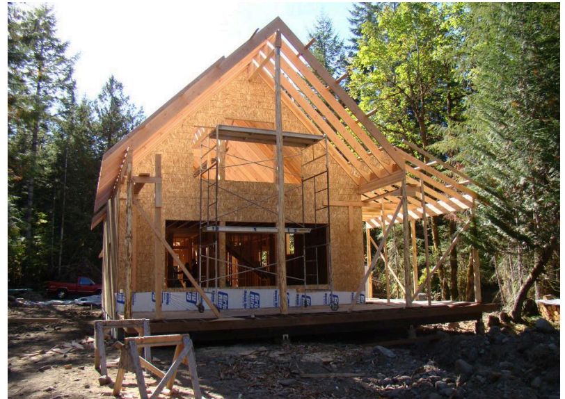
New Construction in Packwood (Photo: Mindy Brooks)
