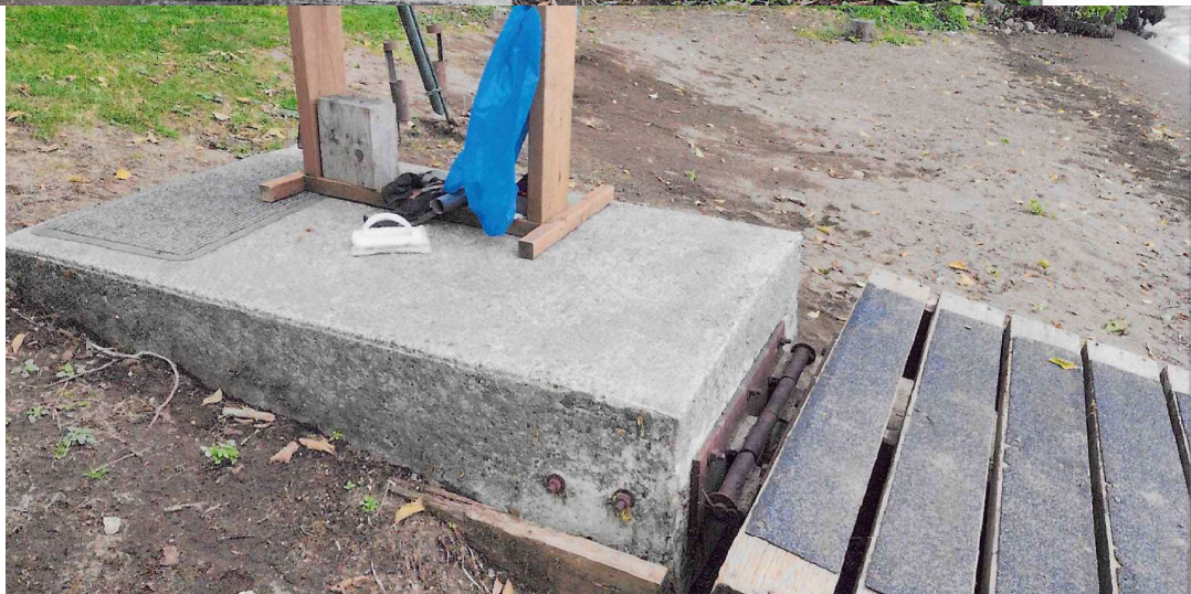
Re-use concrete abutment
