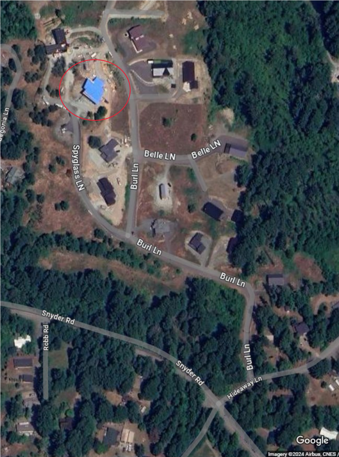
Blue roof is the location of the single family residence under construction on proposed lot 4.
