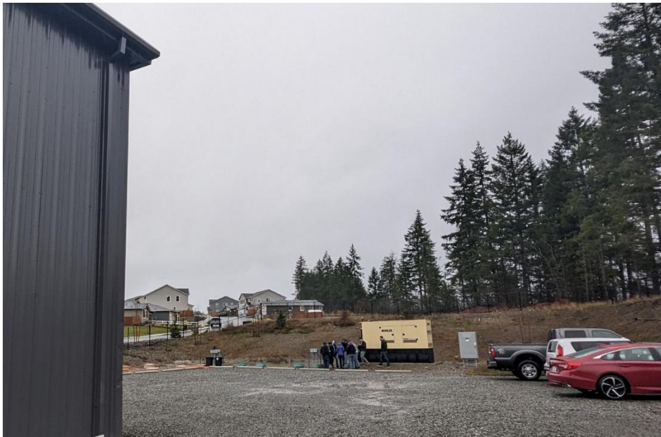
Image 2: View of Holding Tank Areas and Back-Up Generator
