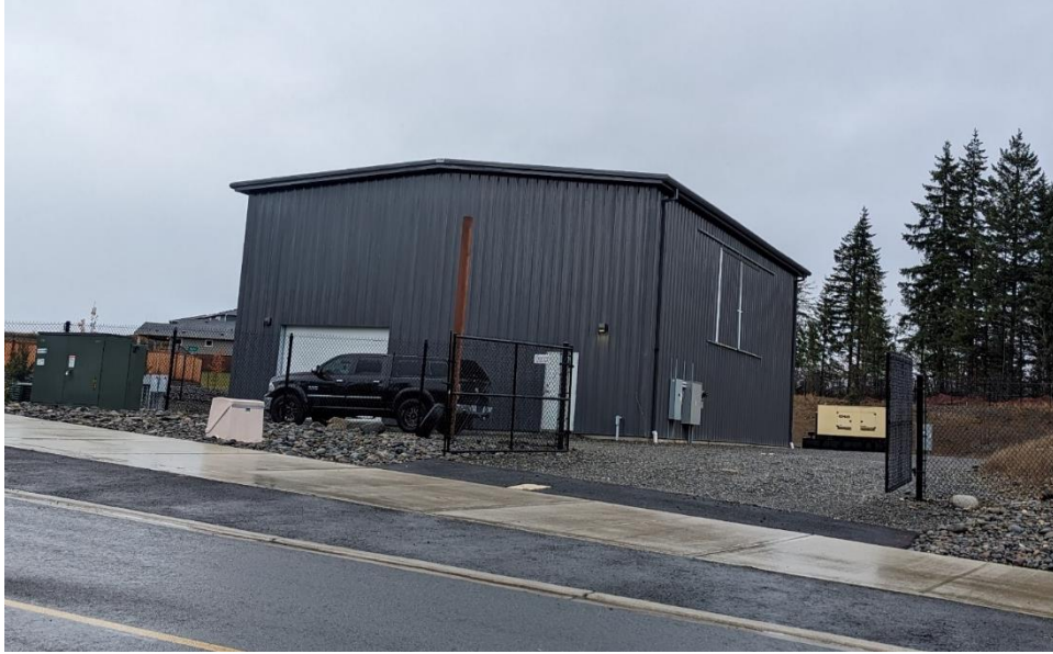
Image 1: View of MBR Treatment Facility
