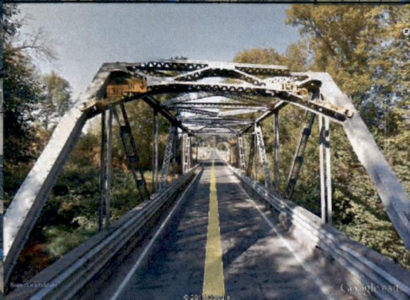
The Ferrier Bridge #93 is a steel truss bridge which was initially erected in 1924 and rebuilt in 1988.
