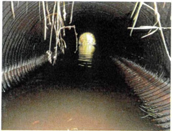
Centralia Alpha Road MP 15.79 inlet
