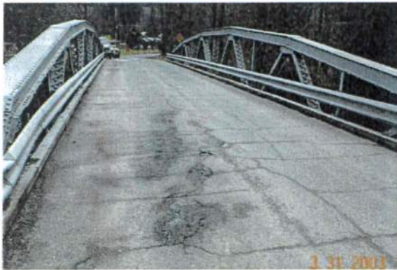
Davison MP 0.01 Bridge #1
