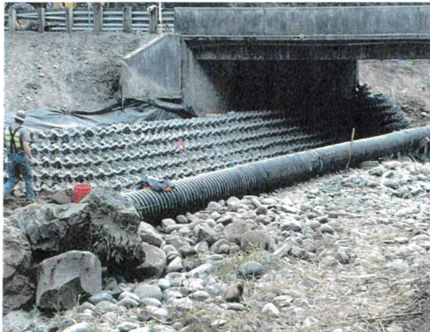
STOWELL MP 0.57, Bridge # 221 Mid-Construction
