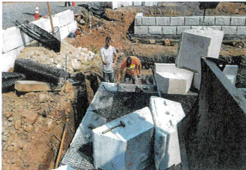
COUSINS MP 3.15, Bridge # 79 Mid-Construction
