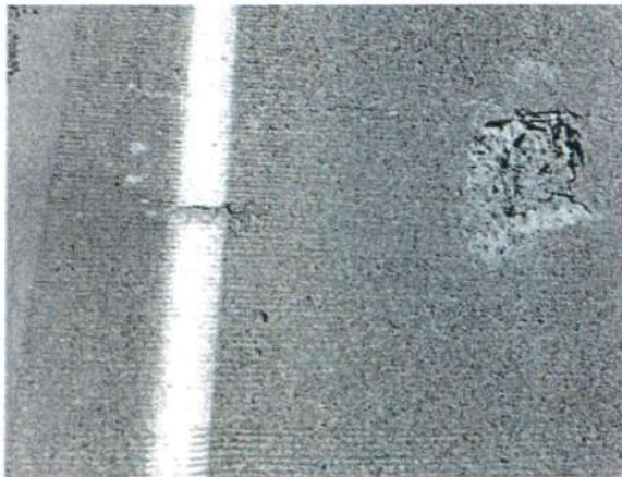
Galvin MP 1.23 Bridge #112
