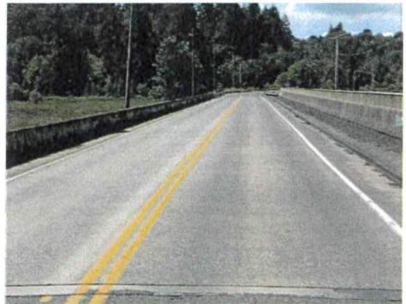
Galvin MP 1.23 Bridge #112
