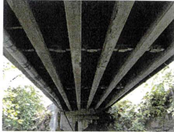
Hinning MP 0.23 Bridge #8
