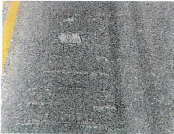
Galvin MP 1.55 Bridge #75
