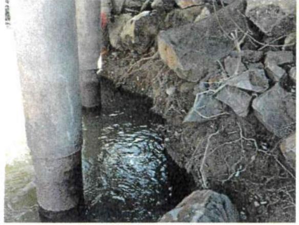
Senn MP 0.89 Bridge #77
