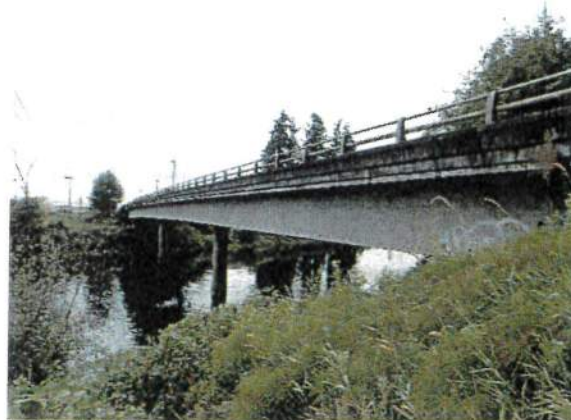
Galvin Bridge #75, built in 1969 is a bridge that requires an underwater inspection every five years.
