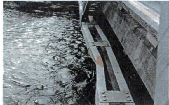
Davison MP 0.01 Bridge #1
