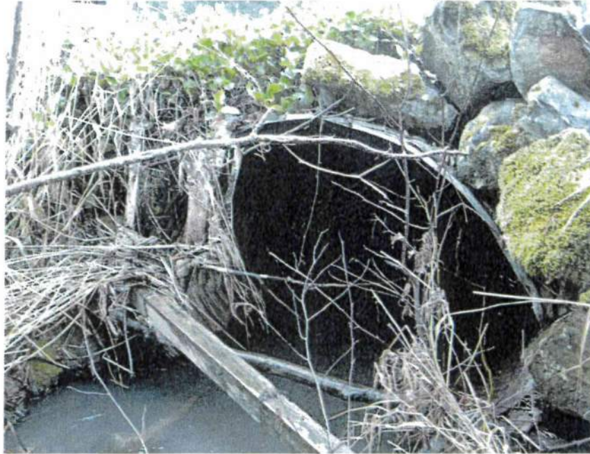
COUSINS MP 3.15, Bridge # 79 Pre-Construction
