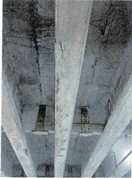
Hinning MP 0.23 Bridge #8
