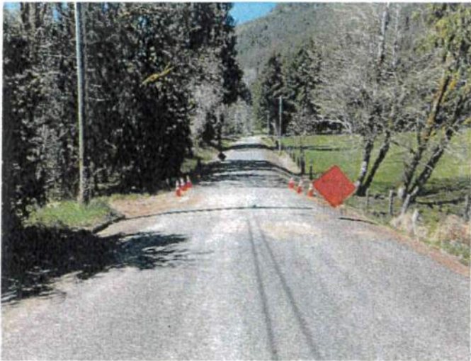
Crumb Road MP 0.17 roadway above culvert
