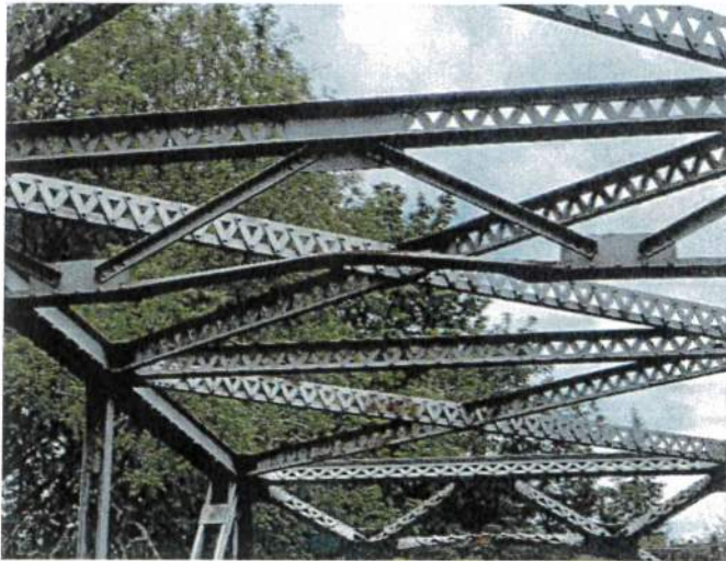
Ferrier Bridge #93 bent cross bracing
