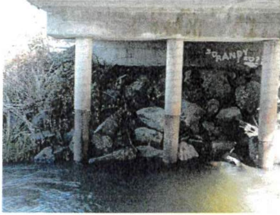
Senn MP 0.89 Bridge #77
