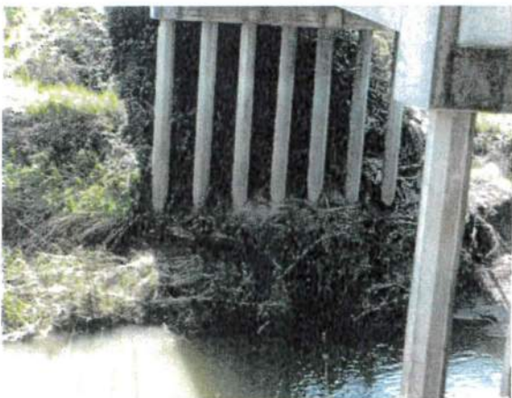
Wildwood MP 10.14 Bridge #3
