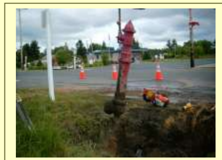
Removal of leaking hydrant.
