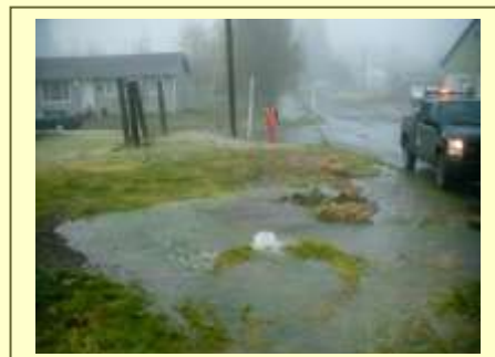
Street conditions from a broken pipe.
